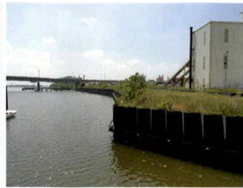
View Toward Project Site and Frederick Douglas Bridge
