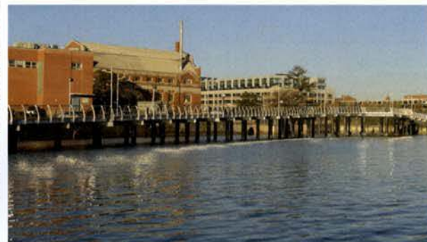
Footbridge between Diamond Teague Park and The Yards
