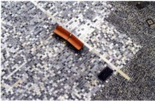
Stone Pavers at Water Feature
